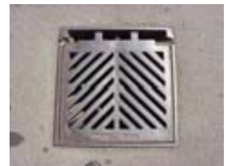
Bicycle-friendly catchbasin cover.
