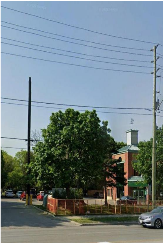
Shrouded Monopole (7828 Kennedy Road, City of Markham)
