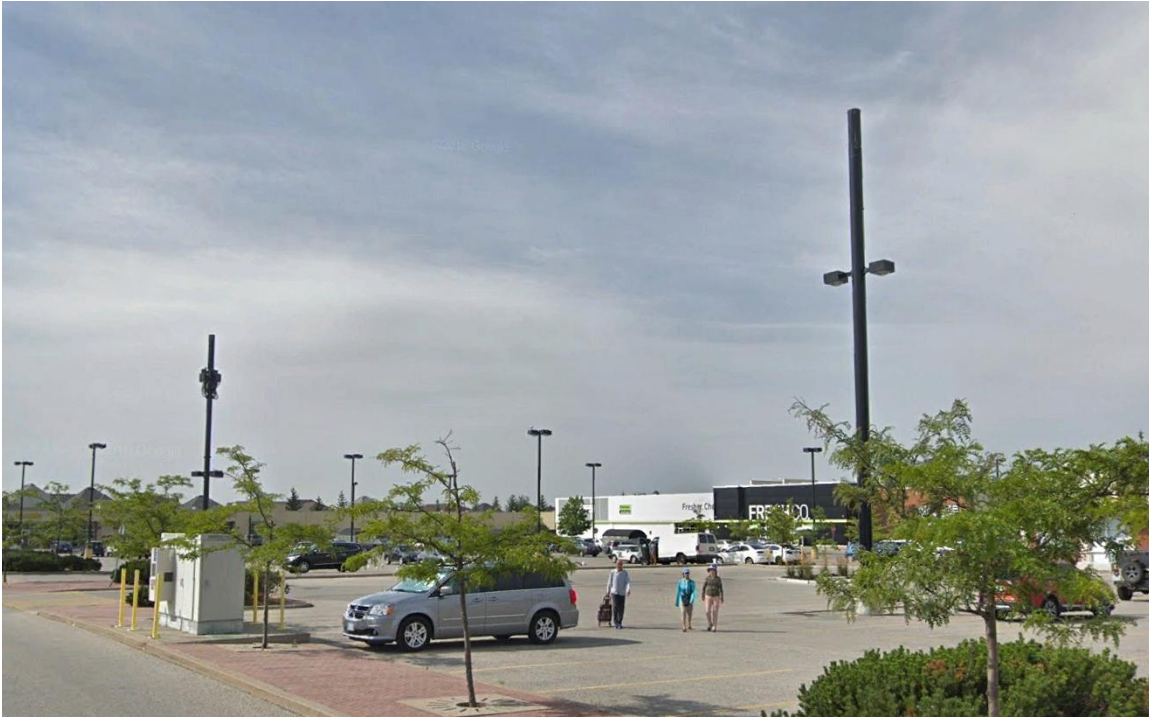
Streetlight Stealth Towers (9610 McCowan Avenue, City of Markham)
