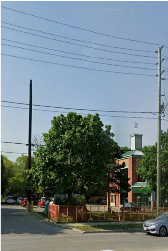
Shrouded Monopole (7828 Kennedy Road, City of Markham)
