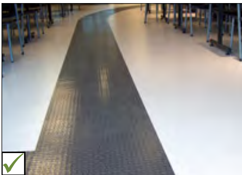
Tactile floor surface to guide users with vision loss.
