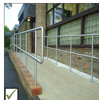
Figure 7c: Handrail Returns to Floor
