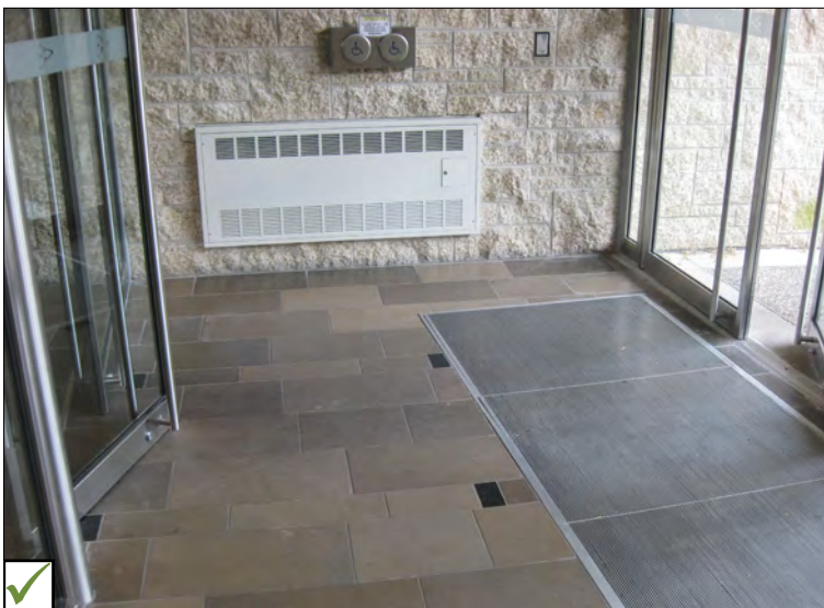
Example of a recessed floor mat system which is preferred.
