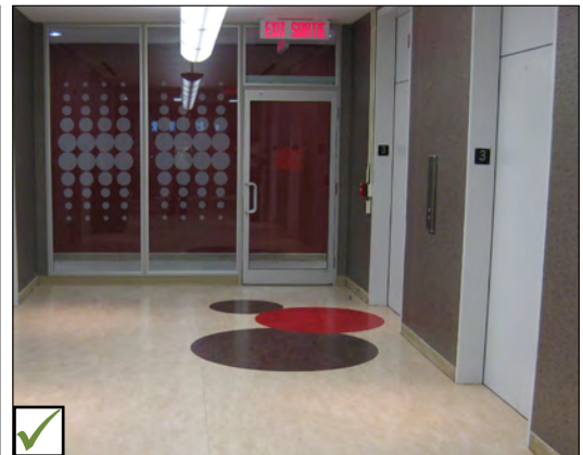
Examples of floor surface and elevator door finishes that minimize glare.
