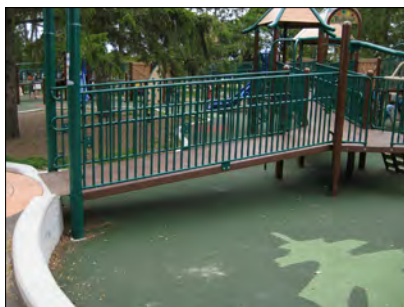
Ramp connected to elevated play components.
