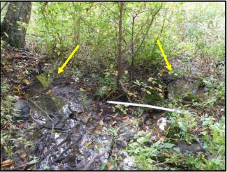
Photo 65 (Location 63) SDF-C. Looking upstream at perched culvert under golf cart path. Note scour pool immediately downstream.
