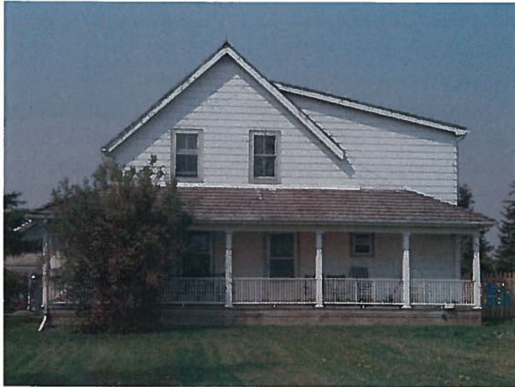
Front (east) View of 10228 Kennedy Road
