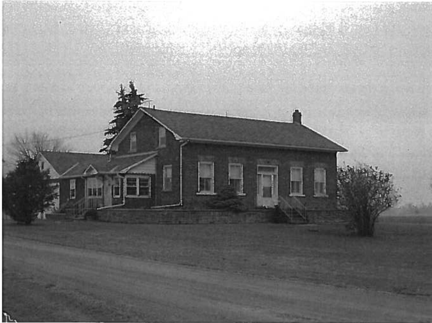
Lyon-Schell-Frisby House East 1/4 Lot 25, Concession 4 3575 Elgin Mills Road East c.1850
