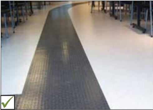
*Tactile floor surface to guide users with vision loss.*
