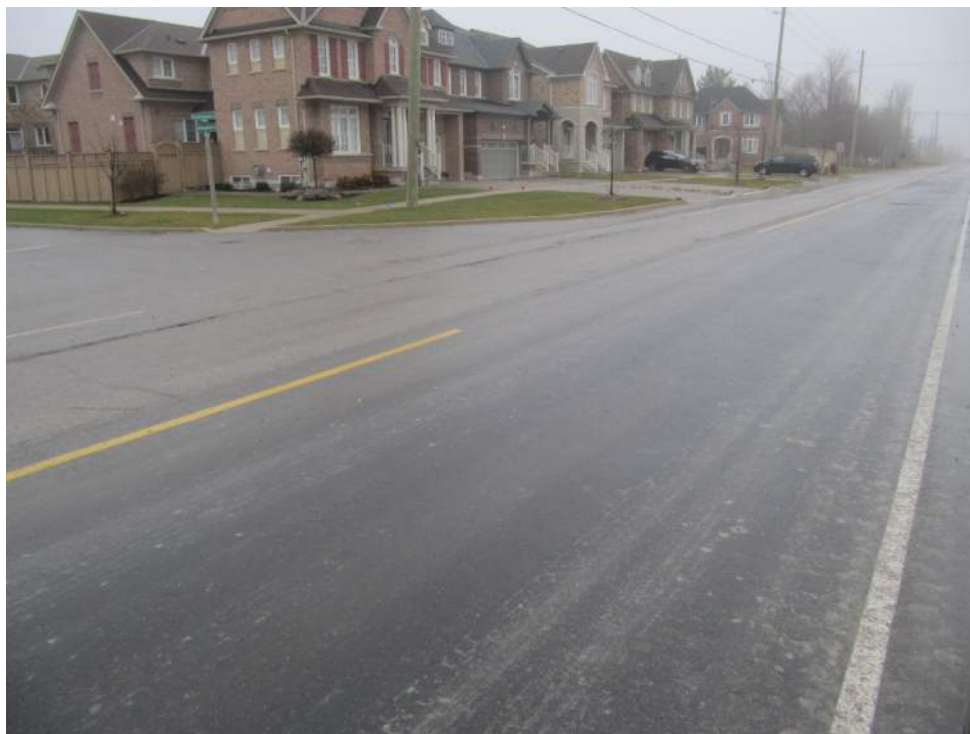
Photo 2: Patching and longitudinal joint deterioration on Victoria Square Boulevard
