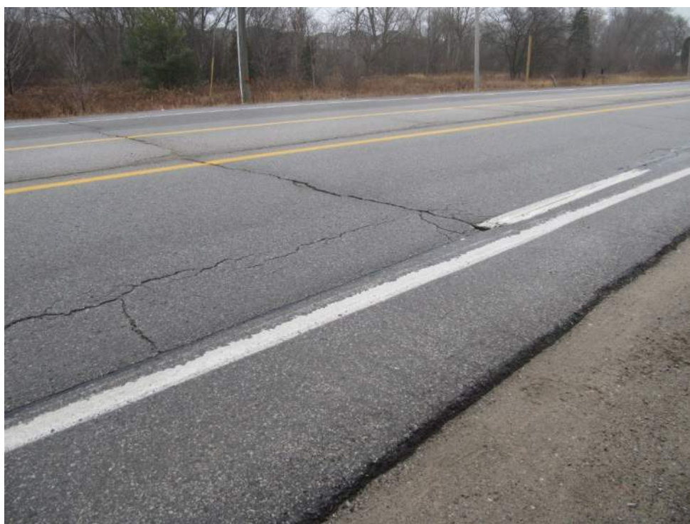
Photo 3: Transverse and fatigue cracking on Victoria Square Boulevard
