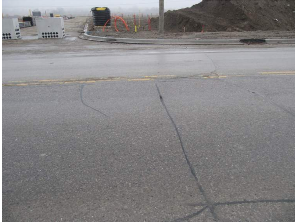
Photo 4: Crack sealing, transverse cracking and longitudinal joint deterioration on Victoria Square Boulevard
