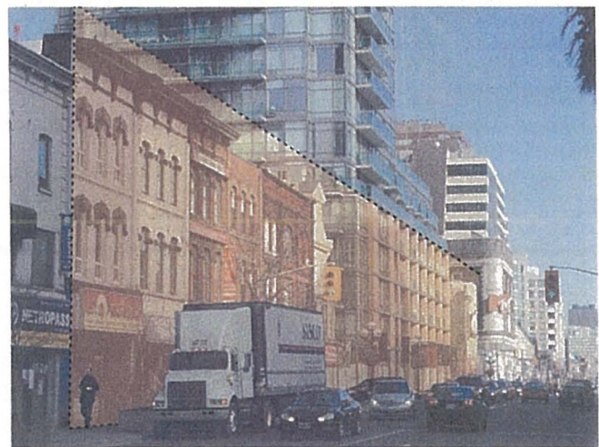
The 18 Yorkville project at Yonge Street and Yorkville Avenue in Toronto is an example of a contemporary point tower. It clearly demonstrates how a high-rise building in combination with a mid-rise base building can fit in by strengthening the street wall, using a small floor plate to minimize shadows and present an elegant profile.
