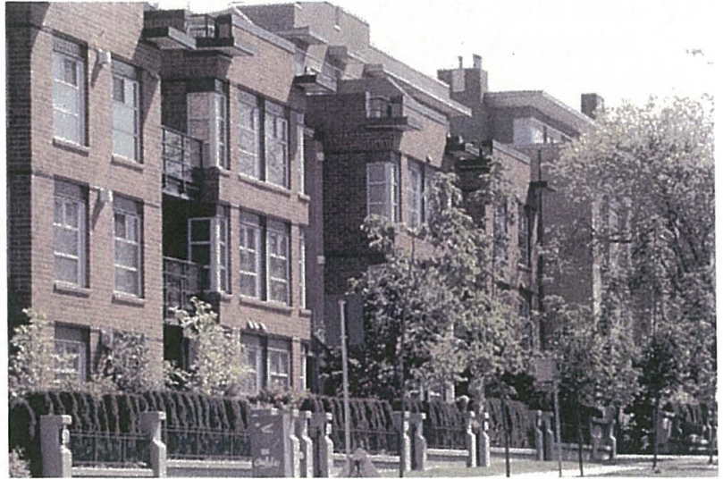
Projections—such as bays, balconies and stoops—away from the principal street wall face will provide variety and allow for individual architectural expression.
