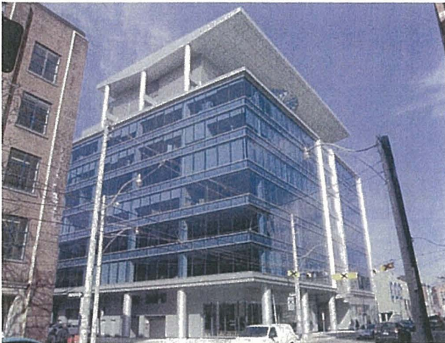
The recently completed headquarters for a software company on King Street East in downtown Toronto is the first LEED®-rated commercial building in Canada (targeting LEED® Silver). By applying sustainable building principles and techniques, the projected energy consumption and cost will be 30 to 50% of a comparable building of typical design. (source: SAS Canada)
