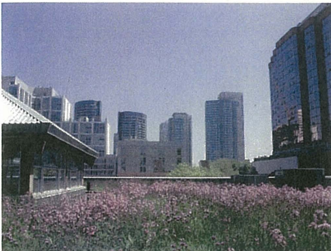
The green roof at Mountain Equipment Co-op in downtown Toronto is one of the flagship projects for the sustainable building movement in North America. All new development within the Yonge-Steeles study area could incorporate similar techniques to reduce runoff, reduce heating and cooling costs, improve local air quality and normalize local microclimate.
