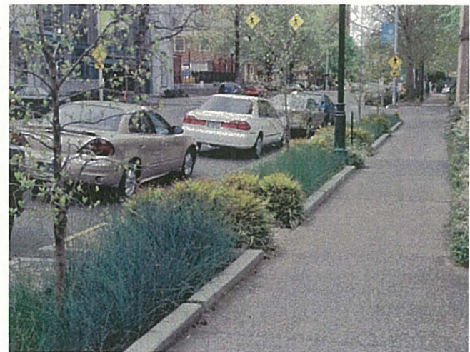
Portland Oregon's Green Streets project makes use of planting areas to help reduce runoff by increasing the amount of permeable surface, thus becoming an important part of the City's green infrastructure. (source: www.sitephocus.com)
