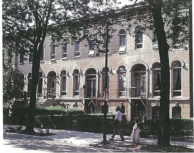
The scale and detailing of the first couple of floors above street level greatly influence the quality and comfort of the pedestrian realm.
